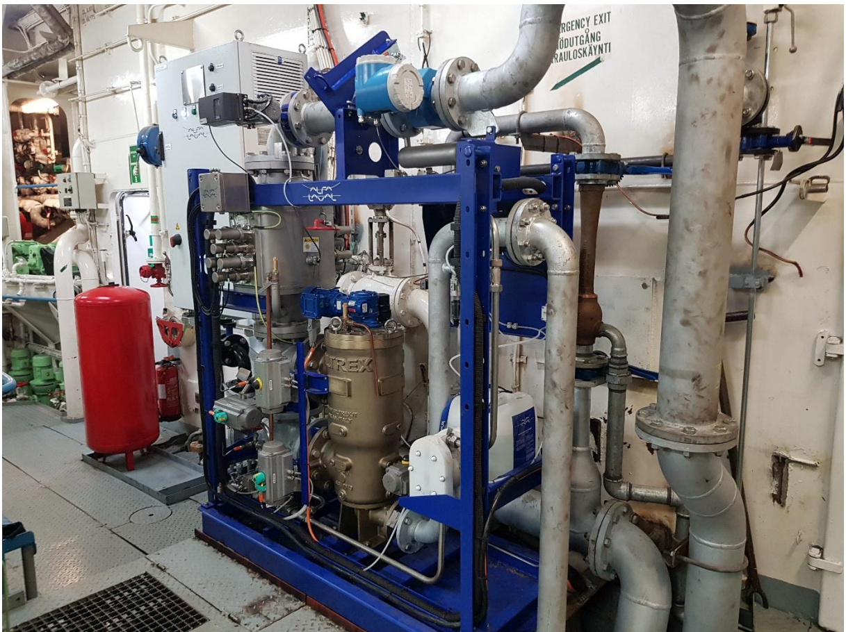
Engine room and ballast water treatment system.
